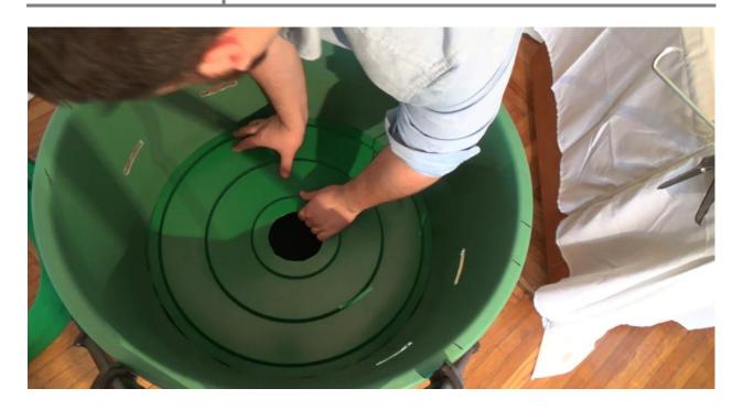
Use sanitary silicone to insulate and glue the cap to the inside of the barrel. Make sure you don't leave any gaps as dust might contaminate the water beneath it.
